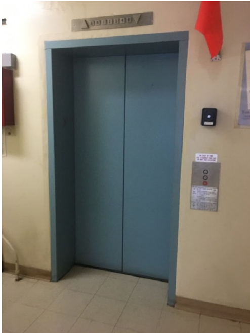
Solids Handling Building Elevator
