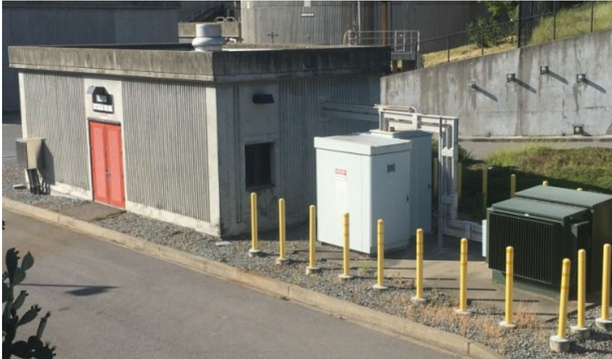
Switchgear building and transformer
