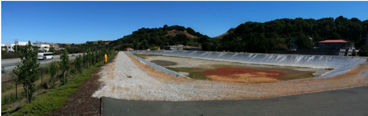
Effluent Storage Pond
