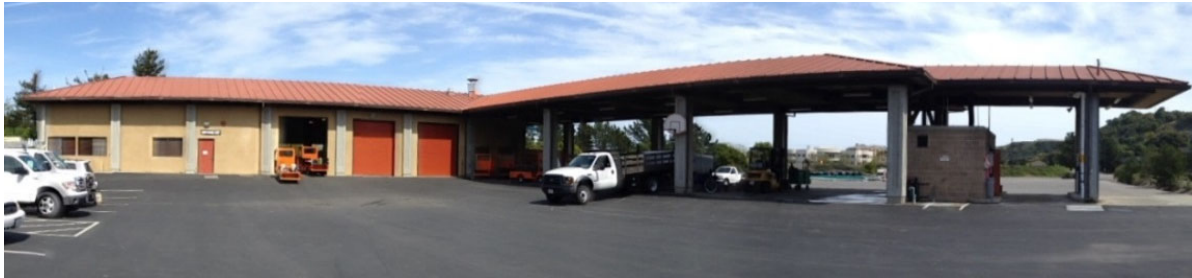
Maintenance Building with standing seam metal roofs
