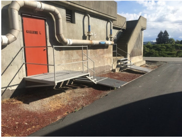
Stair modifications to account for settlement
